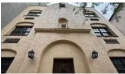
As congregations shrink, church-to-housing conversions take center stage
